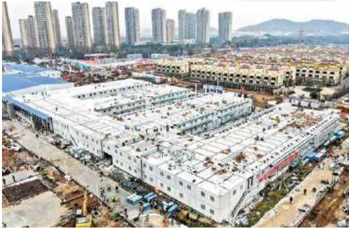
火神山医院 ( Culcan Mountain Hospital )
